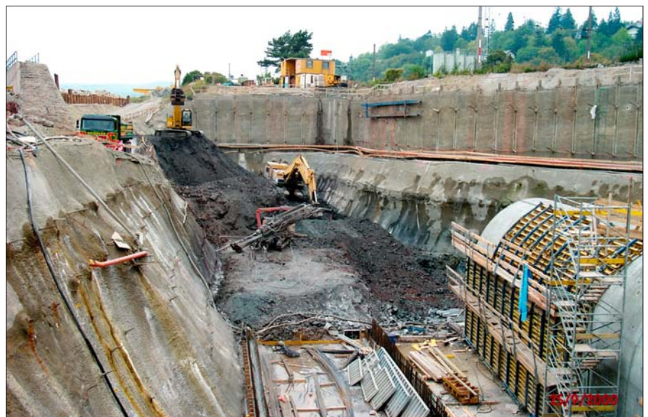
View of the western end of the building pit.
