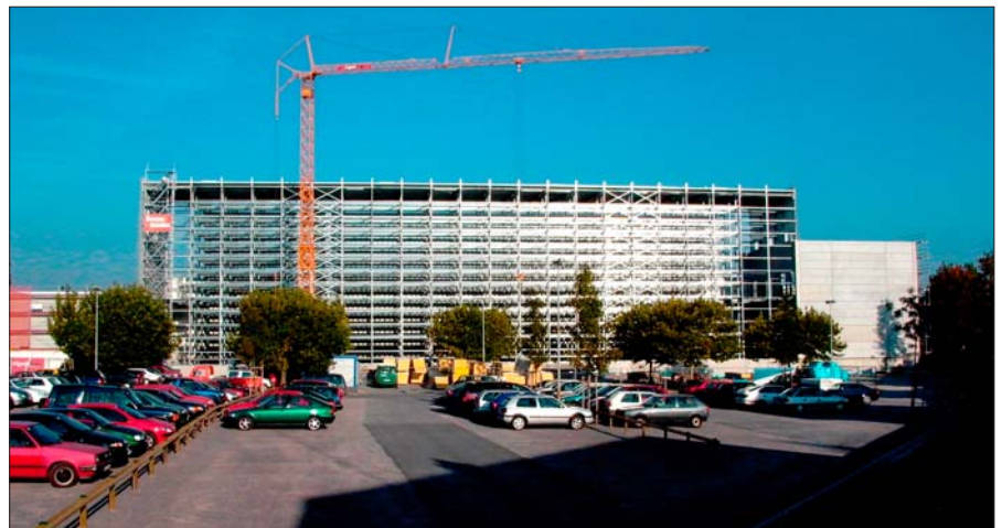
The warehouse during shell phase
