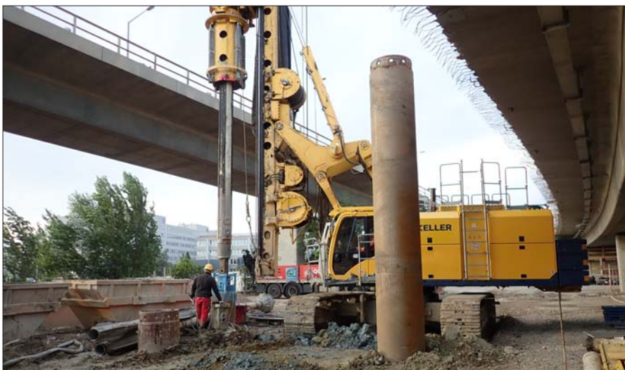
Bored pile works in the area of a bridge enlargement
