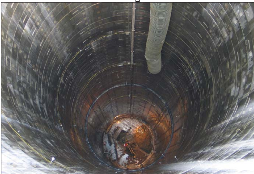
View into the Paierdorf shaft during excavation
