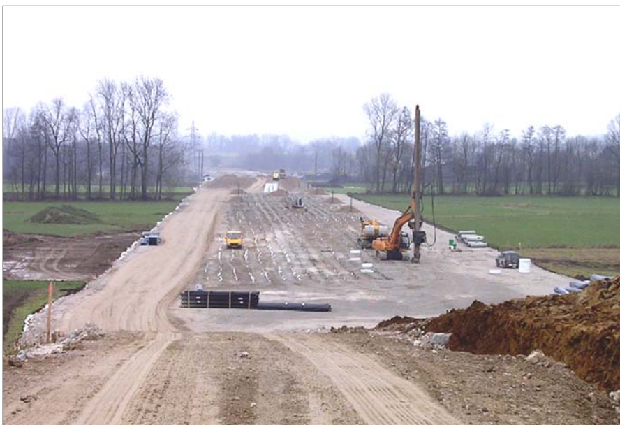
View towards the dam plane during placement of the vertical drains
