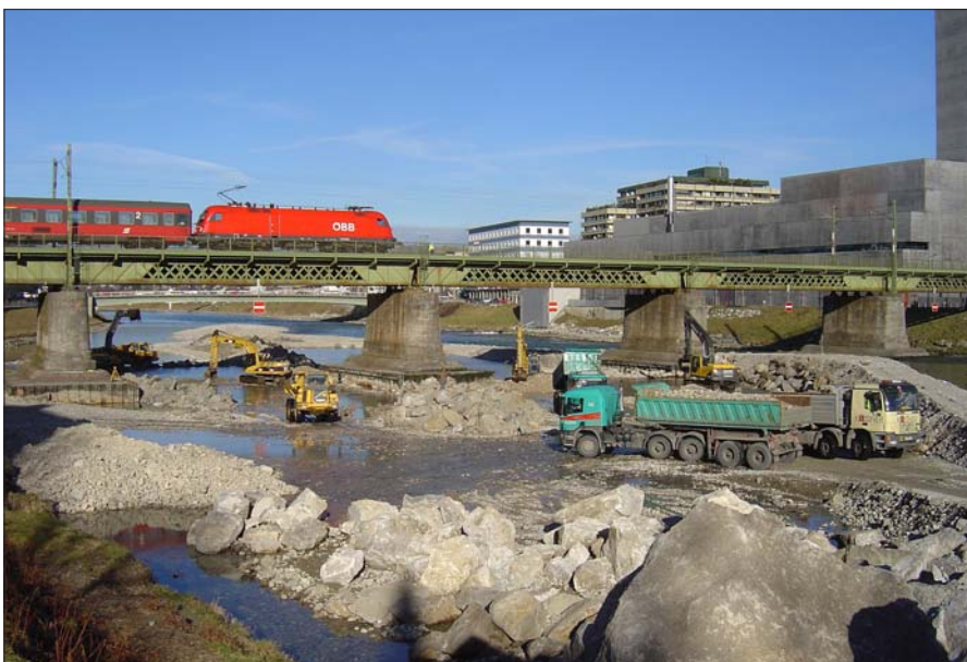
Salzach Bridge, securing of river bed
