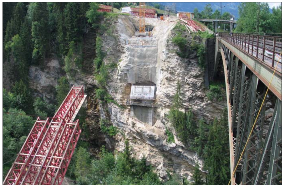
View of the Anger Gorge Bridge, existing and new (under construction); View towards abutment side Schwarzach
