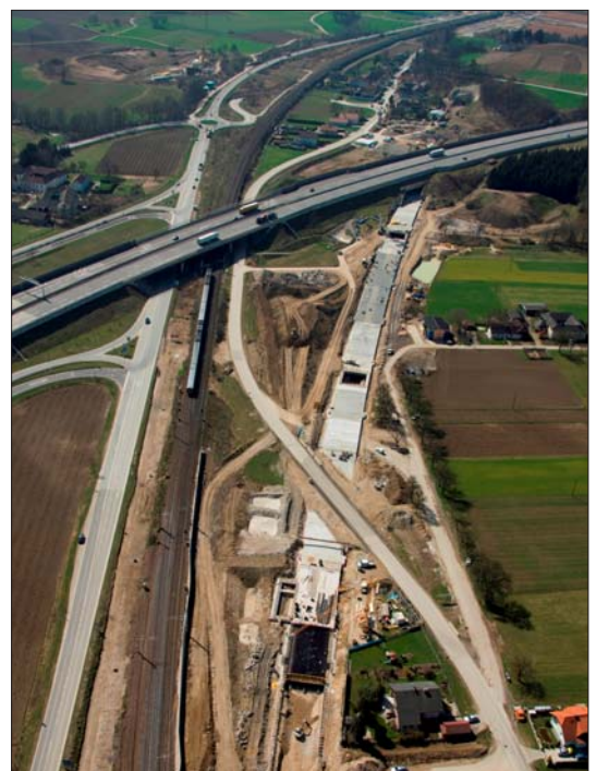
Overview cut-and-cover top-down method
