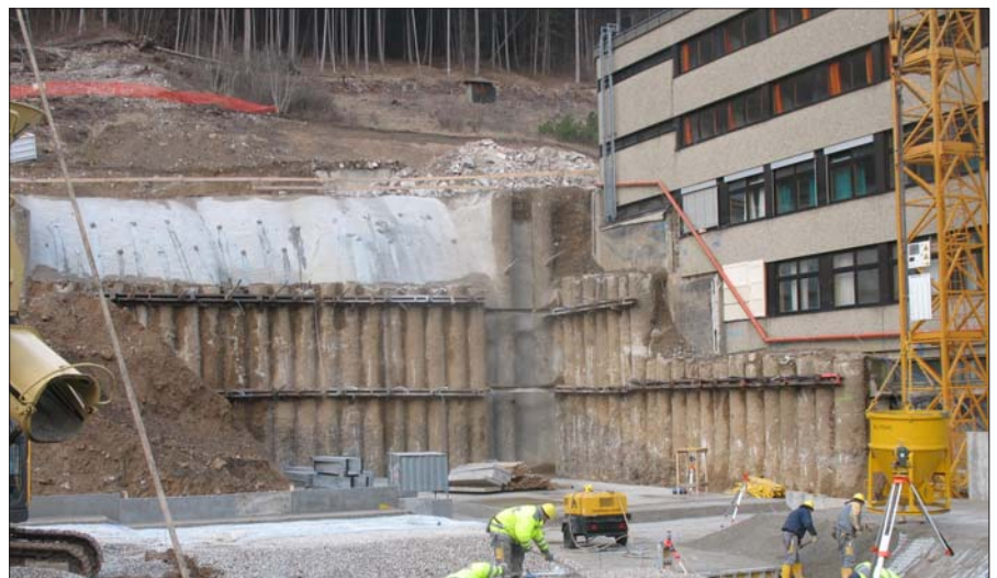
Building Pit Dormitory
