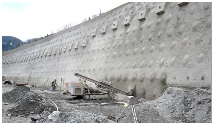
Slope Protection Portal Area Gloggnitz
