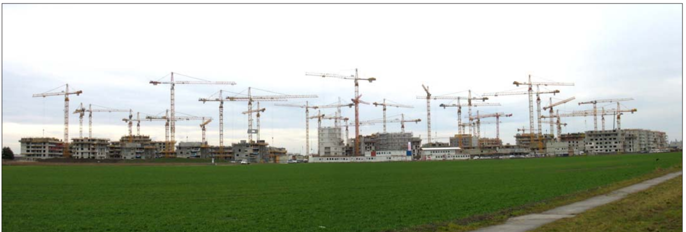
Construction of 20 projects at the same time
