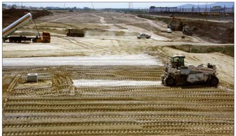
Soil stabilization works
