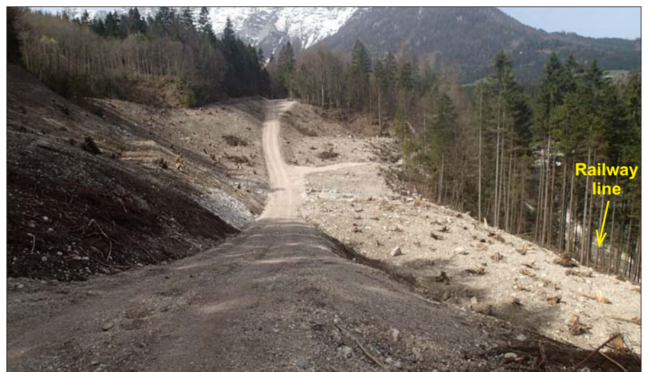
Sliding area after completion of the stabilisation works
