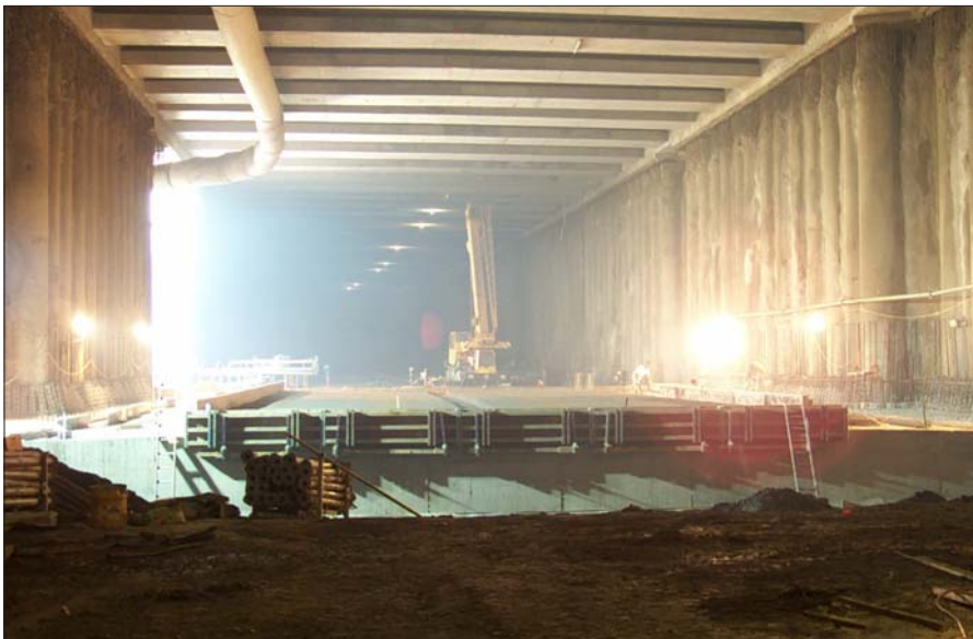
View into the hall during construction of the bottom plate
