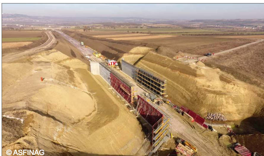
Bridge construction works in the area of the Wildlife Crossing A5Ü40
