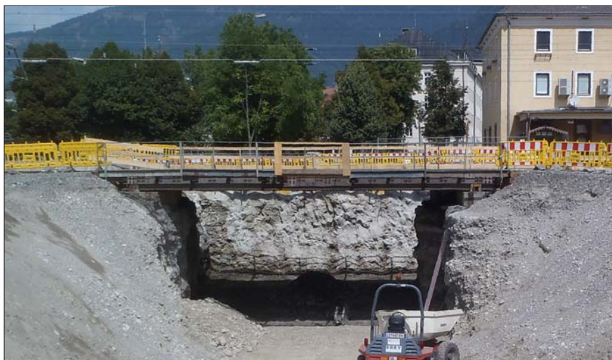
Pedestrian tunnel south: Construction pit support system and foundation of the auxiliary bridges by means of jet grouting
