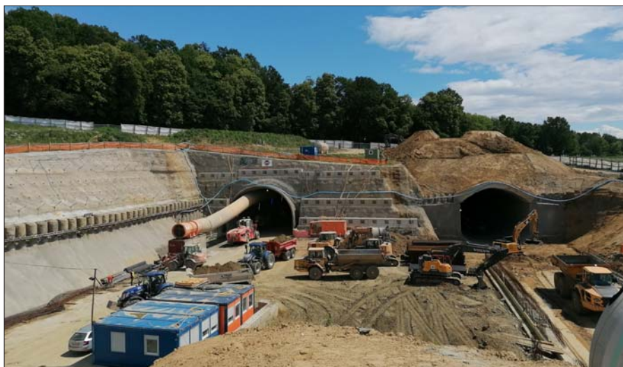
Construction pit support system in the area of the mining portal west and cut-and-cover top-down method at the southern tube
