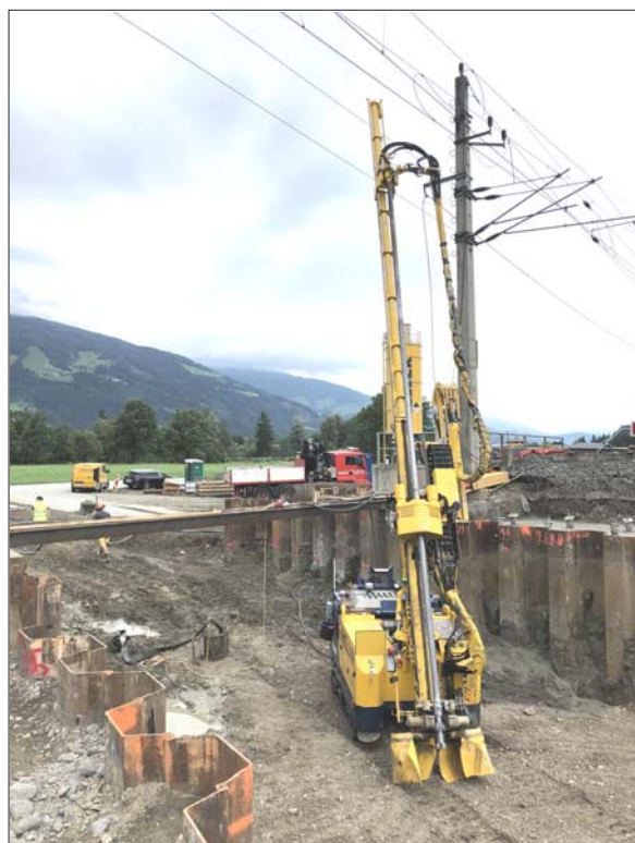
Preparation of the bottom sealing by method of jet-grouting
