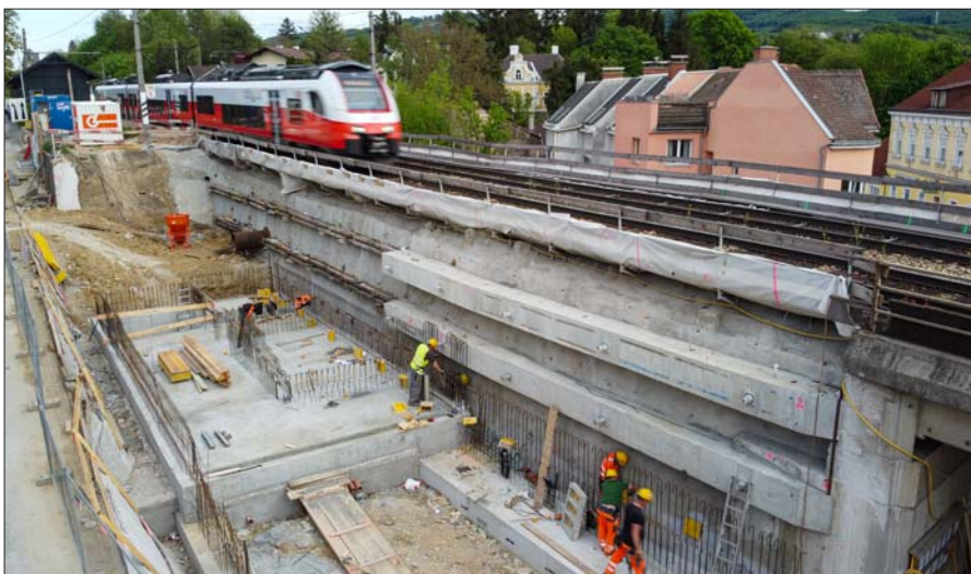
Building pit support system, northern side
