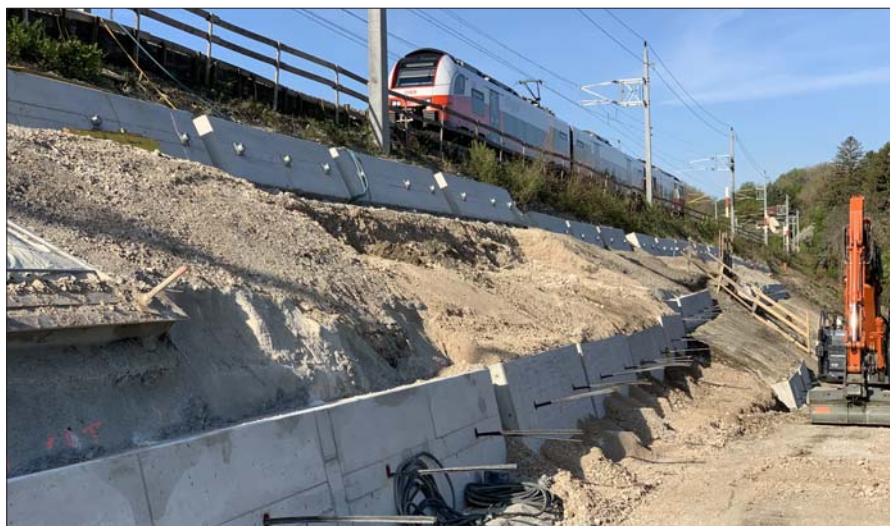
Anchoring works in the area of the embankment reinforcement between km 27.99 and km 28.33 (right side of line)
