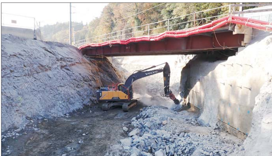
Road underpass, Rock excavation below auxiliary bridges
