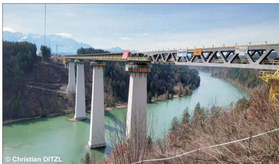
Slide-in of the steel structure (old and new structure visible)
