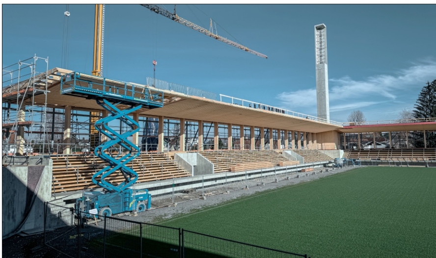
Construction of the eastern stand (in the background floodlight tower South-East)
