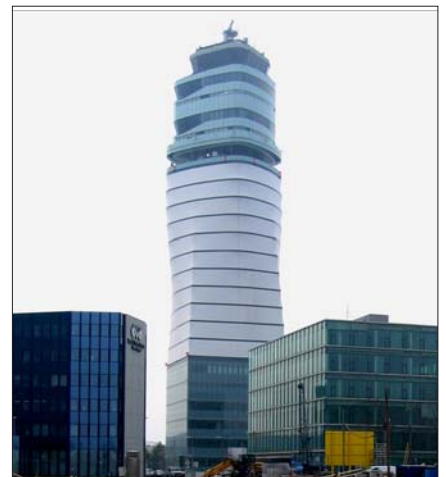
Control tower after completion
