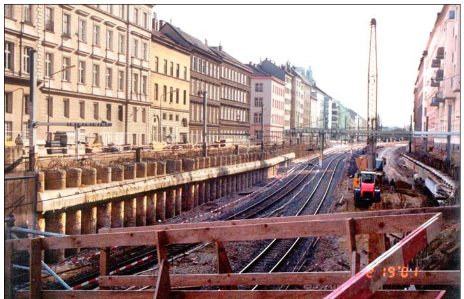
Construction pit at an intra-urban location (view towards south-east)
