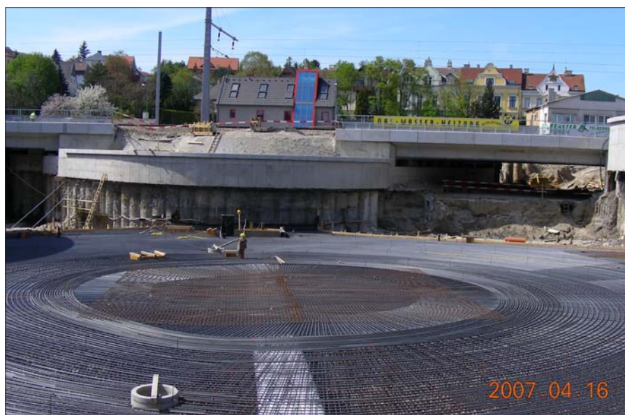
View of the roundabout Aufeldgasse (Below groundwater level); Reinforcement of the bottom plate for reasons of uplift control
