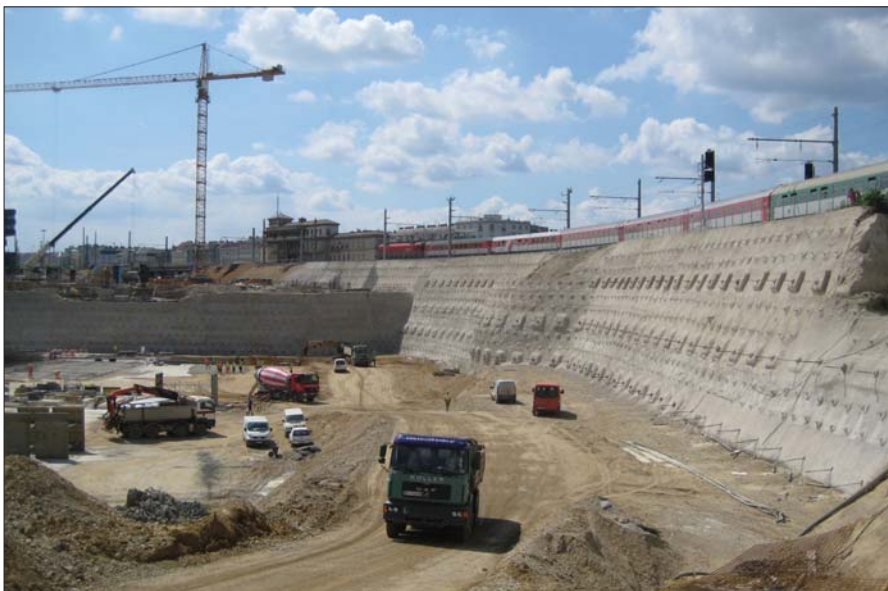
View into the building pit, southern station complex
