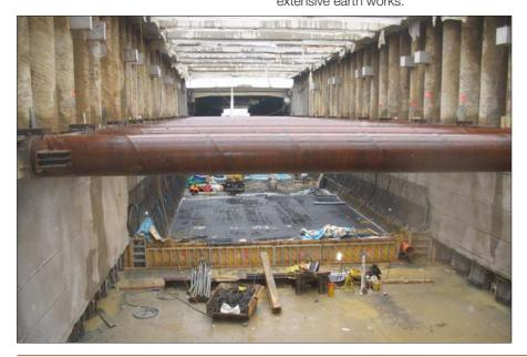
Cut-and-cover Hengsberg South (Area with arch section): Building of base plate under protection of bored pile walls with temporary bracing
