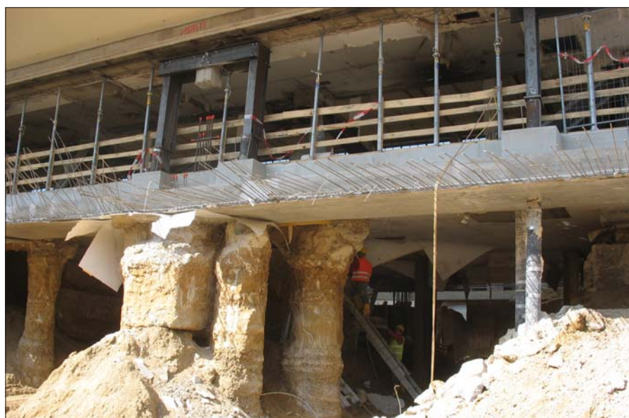
Establishing of basement below station hall; temporary support by jet grouting pillars
