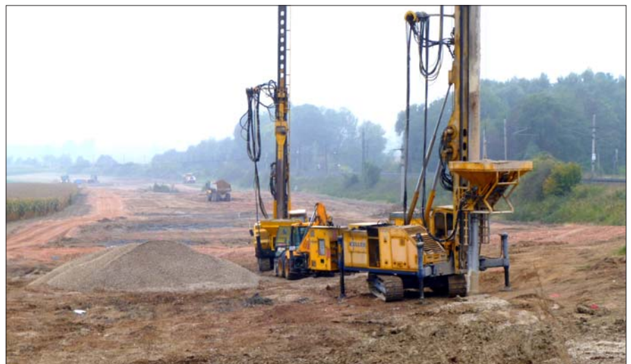
Vibro-displacement in the Area of the Schwaiger Brook Floodplain
