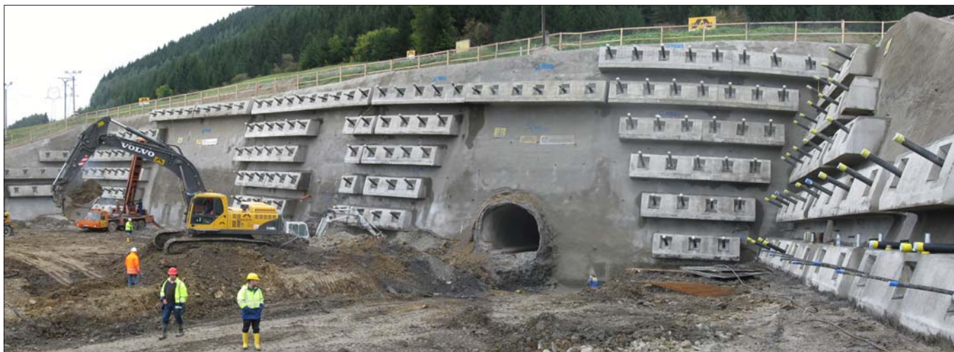
View of the retaining structure at the portal Višňové West
