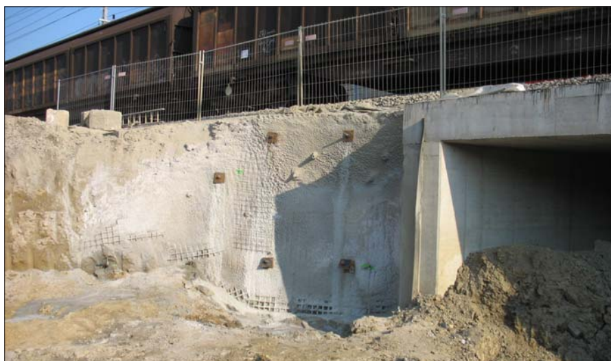
Shotcrete wall with soil nails in the area of the underpass Neilreichgasse
