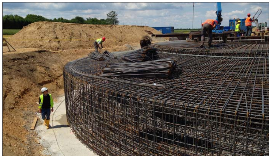
Construction of foundation
