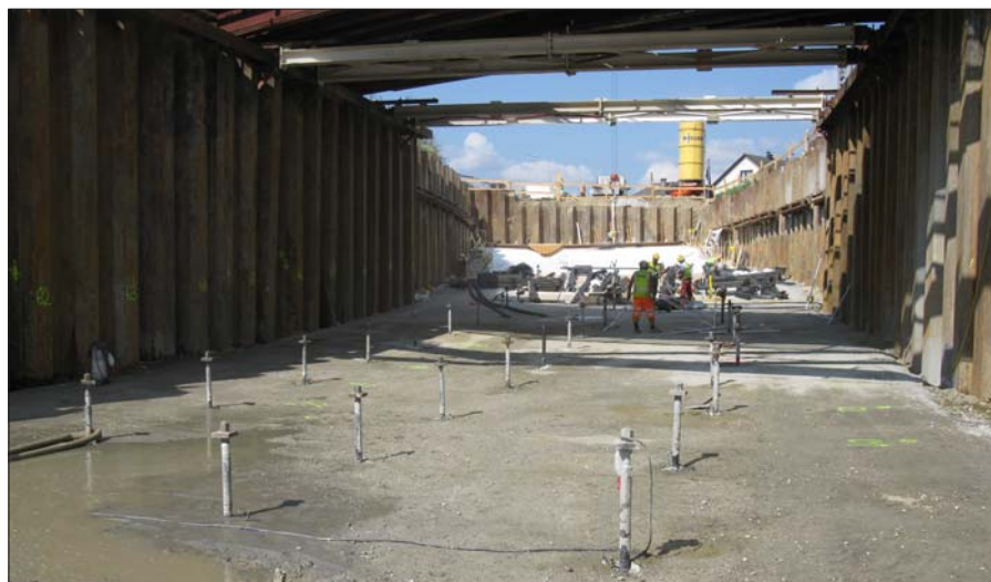
Building pit after construction of the micro bored piles for buoyancy control
