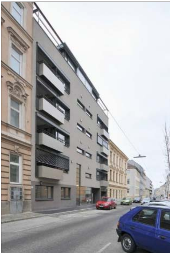
View towards the front of the building at Blumengasse
