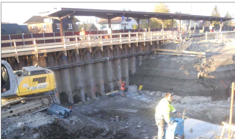
View into the building pit of the pedestrian underpass
