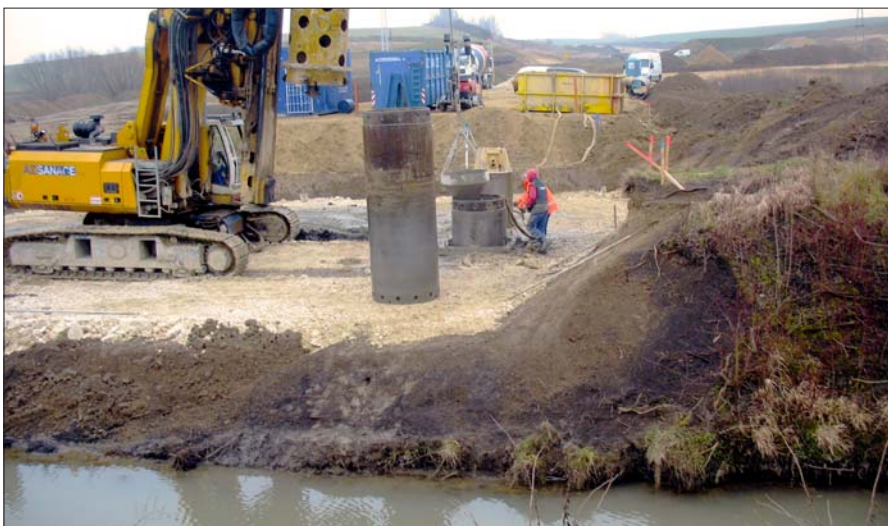
Bored pile works close to a surface water body
