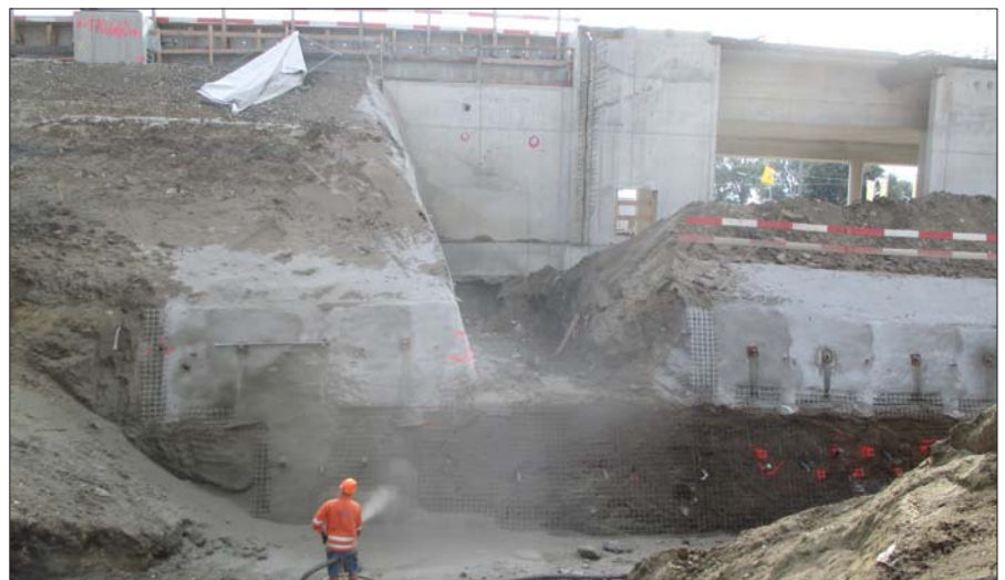
Setting up of the shotcrete wall above the cistern
