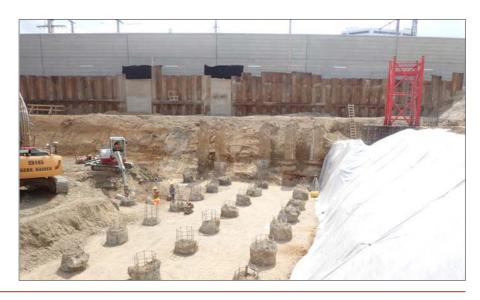
View into the building pit with uncovered foundation piles; In the background the retaining wall towards the railway station
