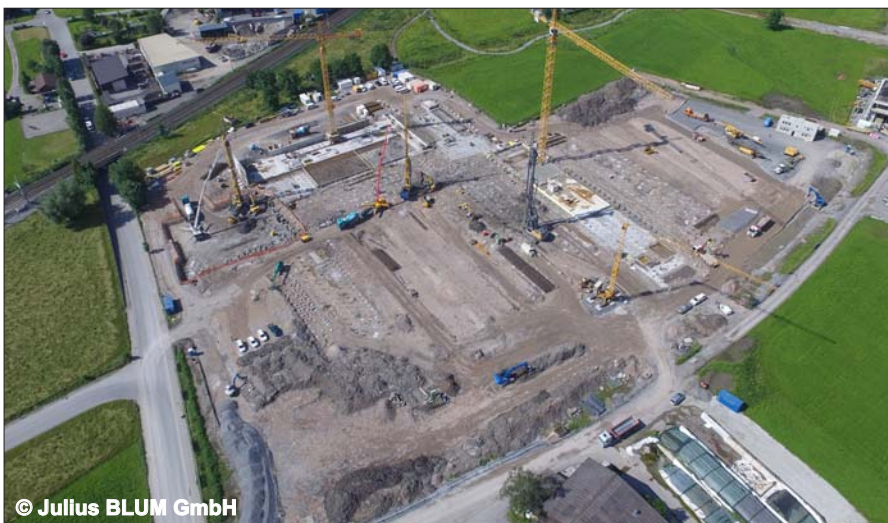
Construction site during pile works; Simultaneous operation of three CFA units
