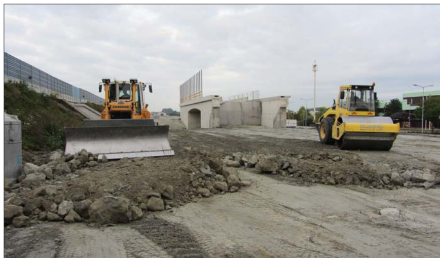
Earth works at the embankment section
