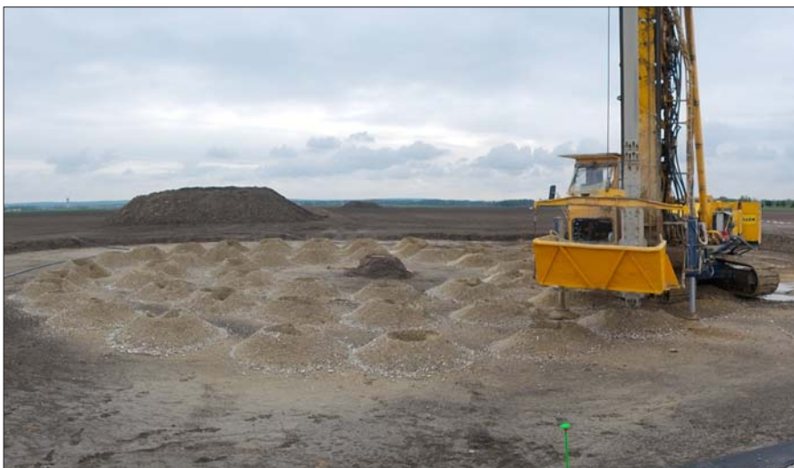
Underground improvement works
