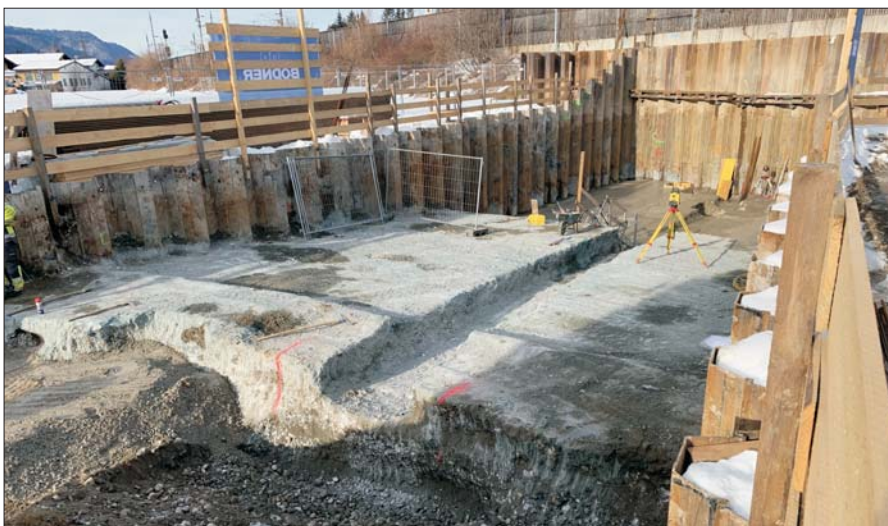
Construction pit Ramsl Road, side southwest with exposed jet grouted bottom
