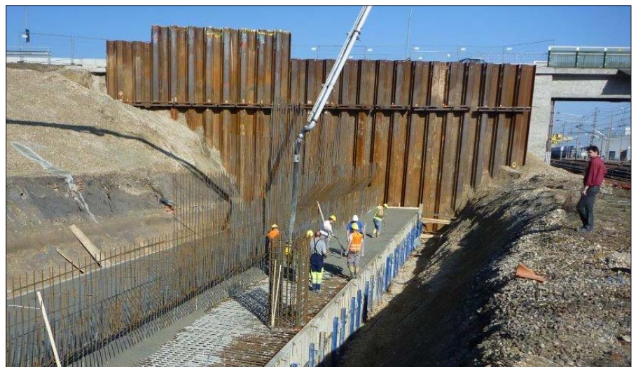
Sheet Pile Wall Reich Bridge, Northern Abutment
